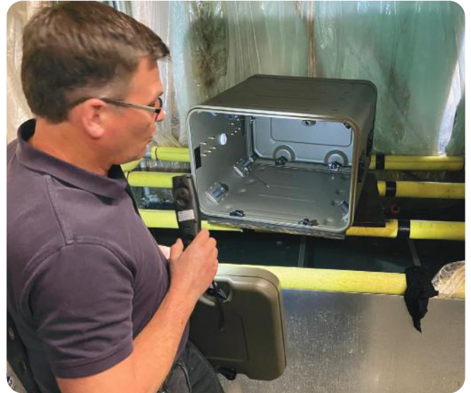
Internal inspection after water test
